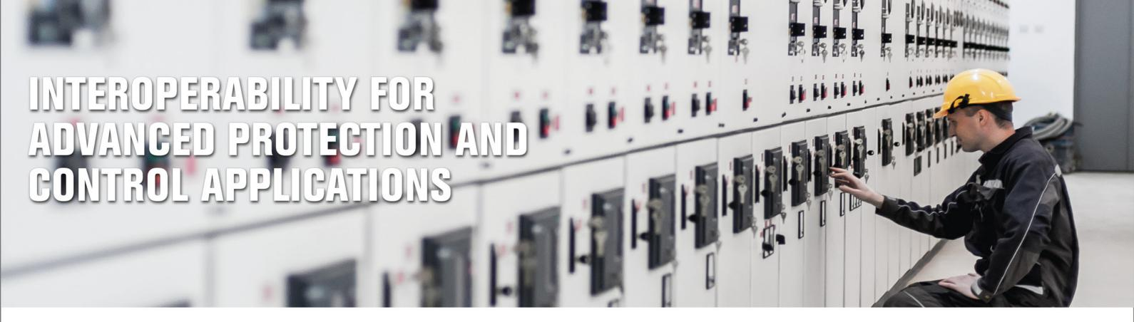
**IEC 61850** is the international standard for communication in substations. It enables integration of all protection, control, measurement and monitoring functions and additionally provides the means for high-speed substation protection applications.
